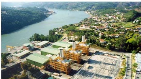
< Turbogás natural gas-fired combined cycle power plant >
