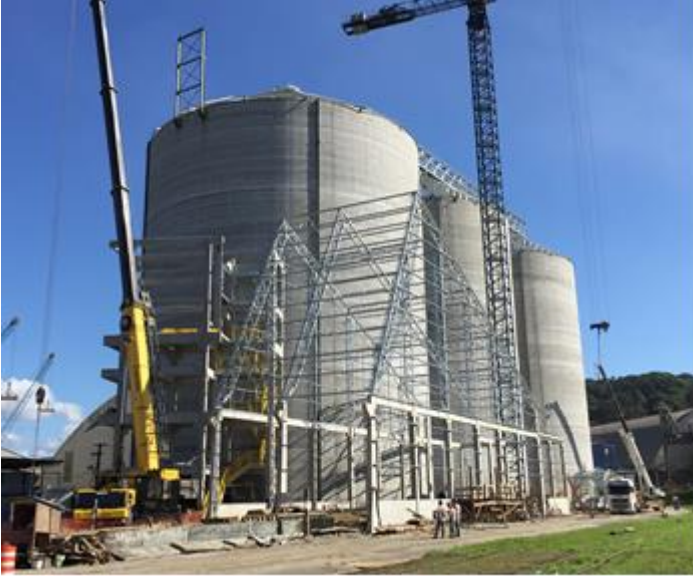
New grain silos under construction
