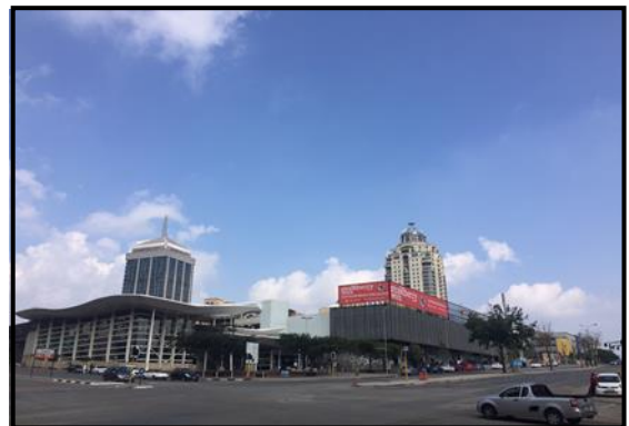
Picture 1: View of shopping mall and Sandton Station which is located in front of Marubeni's Johannesburg Office
